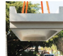
Above: Precast panels at the Global Change Institute made using Wagners E-C Right: Waste clay at a quarry with potential for use as calcined clay
